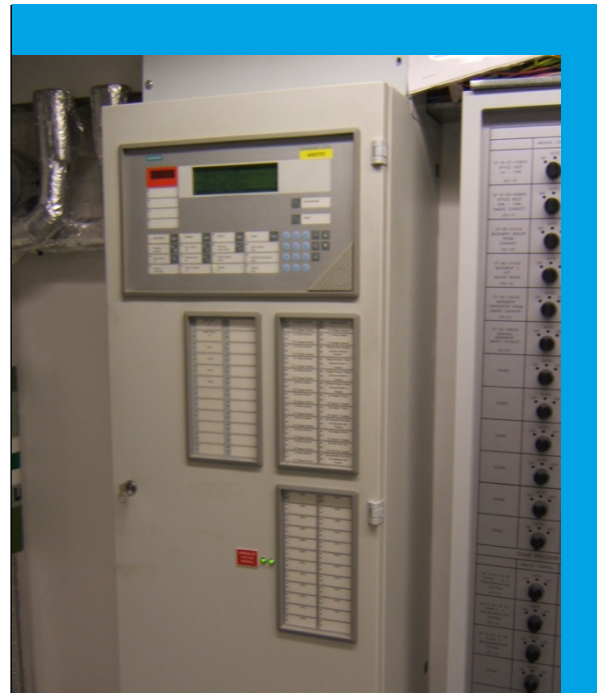
Typical automatic fire alarm panel
